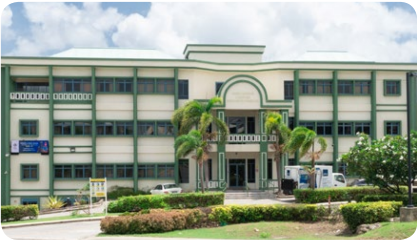
Owen Arthur CARICOM Research Complex
