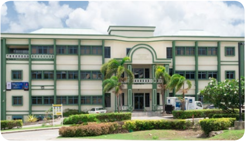
Owen Arthur CARICOM Research Complex
