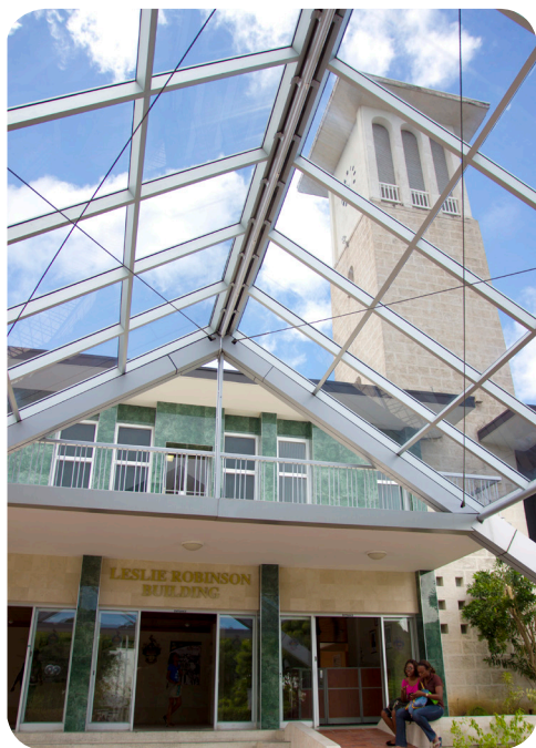
Leslie Robinson Building
