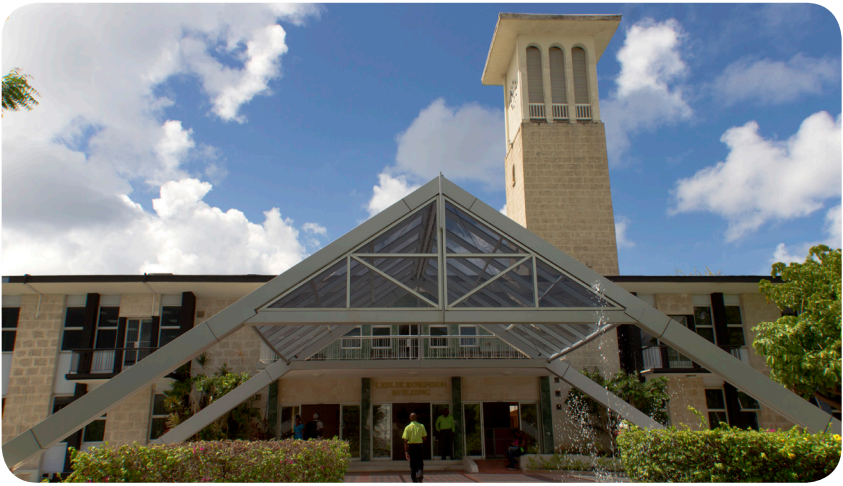
Leslie Robinson Building
