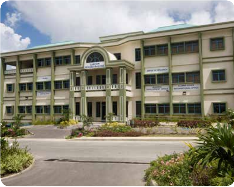
CARICOM Research Building (Map CARICOM PARK Ref 37)
