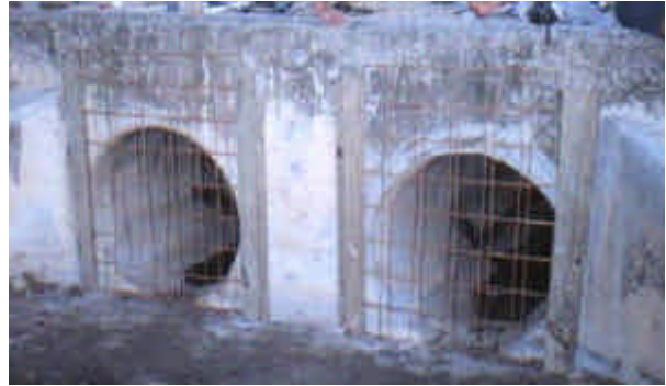
Figure 10. Completed debris traps on the culvert
