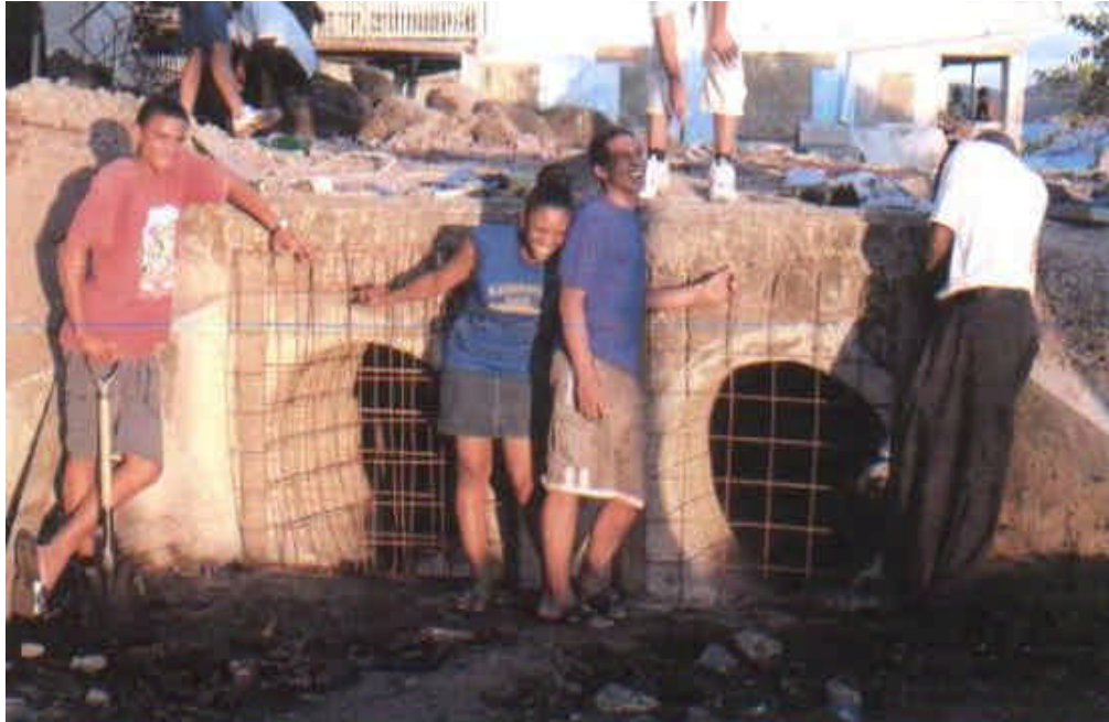
Figure 8. Students working on the construction of the debris traps
