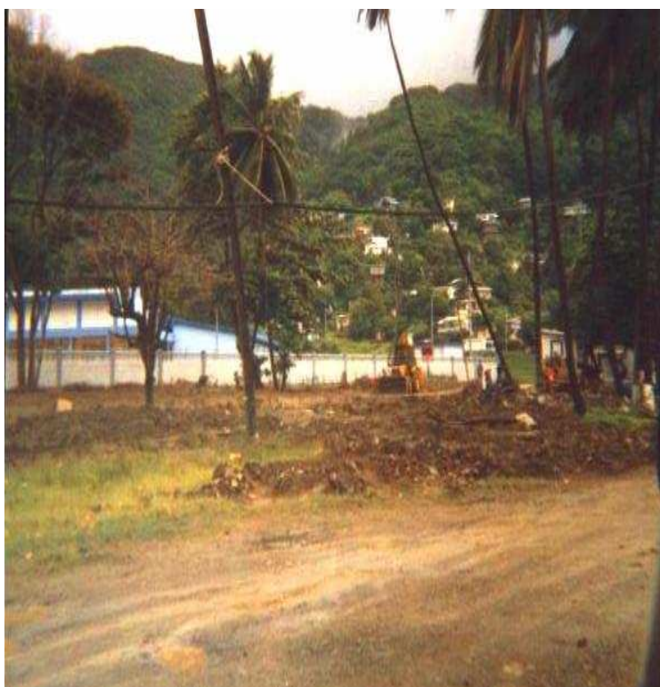
FIG 13: NEW SECONDARY SCHOOL BEING CONSTRUCTED ON THE BEACH FRONT AT SPEYSIDE
