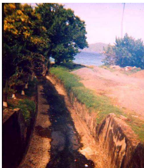
Fig 27: Construction material in piles next to a drain leading to the sea.
