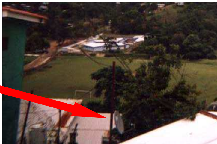
Fig. 24 DirecTV satellite dish commonly noted on houses in Speyside.
