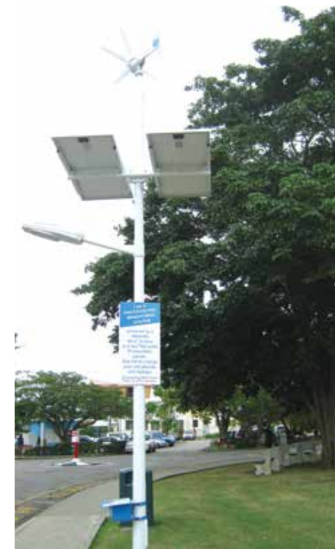
One of the energy saving street lamps at Cave Hill Campus.
