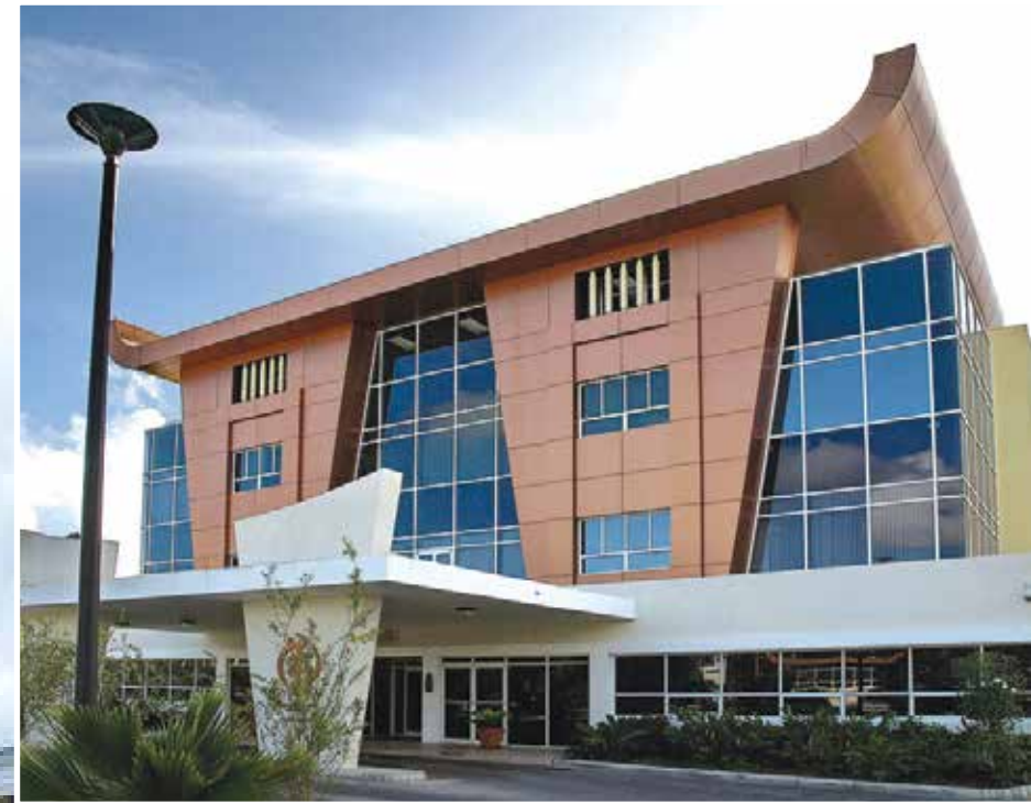
New administration building Cave Hill Campus.
