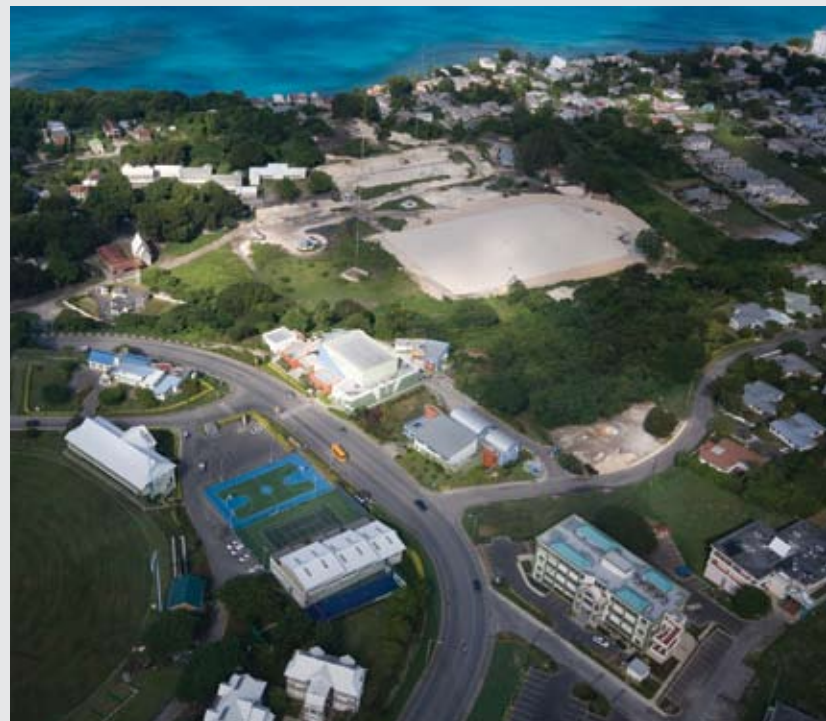
Cave Hill Campus new development at Paradise Park
