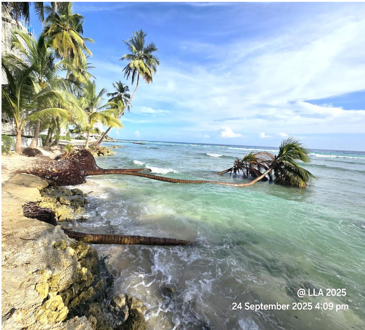
Coastal erosion along the shore near Bridgetown , highlighting a growing challenge for many Barbadian communities as climate stress and shoreline instability threaten livelihoods, infrastructure, and coastal ecosystems. (St. Michael, Barbados, 2025).
