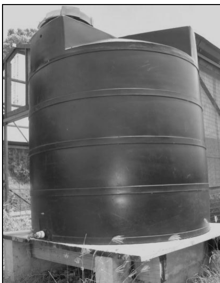
Figure 4.3: Rainwater is harvested and stored in water tanks such as this one on Palm Island
