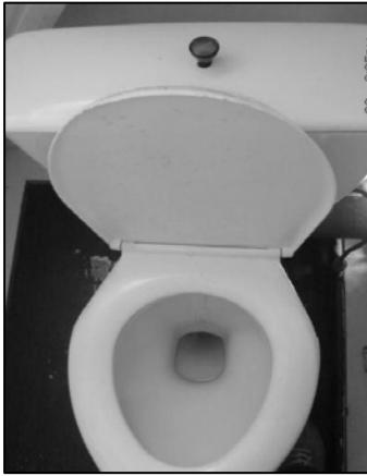
Figure 4.5: A low flush toilet with the low flush device at the top of the tank
