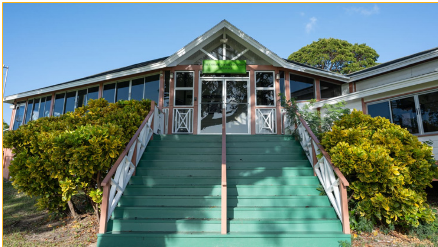
The renovated Staff Lounge
