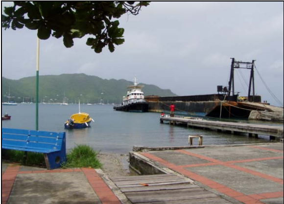
Figure 3.2: Docking facility, Port Elizabeth, Bequia
